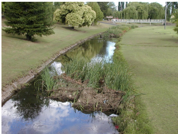
Dumaresq creek can become partially blocked at times (photo taken in 2002). This is still the case in 2017!
