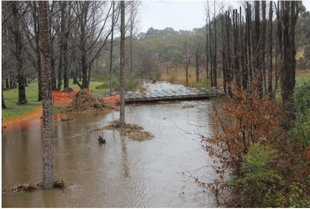
View to the west of the road bridge over Elm Drive at UNE showing an expanded view of water during a flooding event in August 2016
