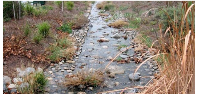
Image: Planting and rock ground treatment of modified creek channel
