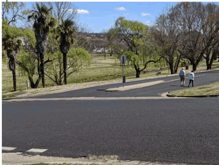
Lack of footpaths in east-west direction (intersection Kirkwood & Faulkner Sts)
