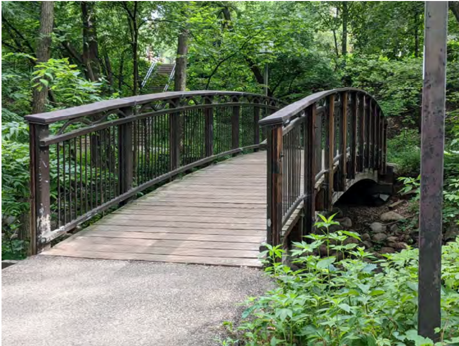
Figure 12: Example of a small pedestrian foot bridge that could span Black Gully.
